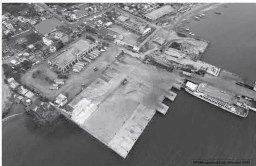
The PPA went on overdrive to start and/or complete various port projects during the last six years of the Duterte administration, including Matnog port (above photo) and other ports on this page.
