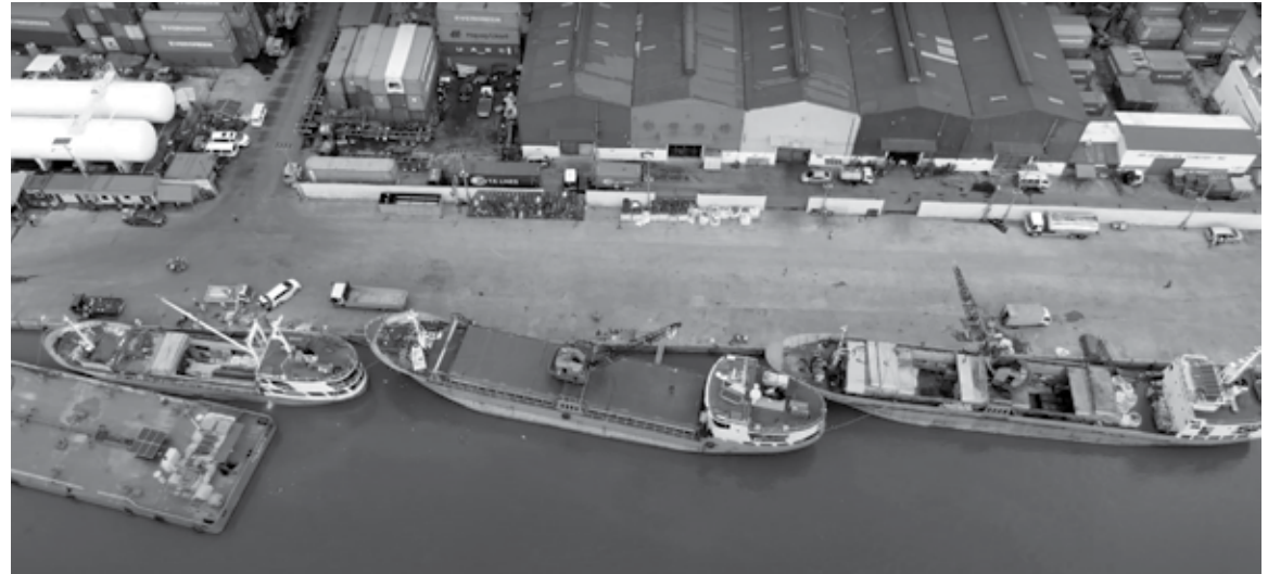
Completed wharf widening project of TMO Pasig Wharf in 2020. Screenshot from PPA Port Construction and Maintenance Department's video.
