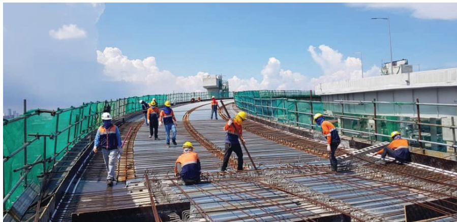
Workers at the Harbor Link construction site. Photo from nlex.com.ph
